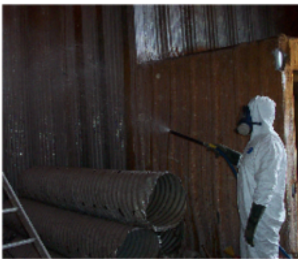
A pressure washer spraying hot water and detergent is a very effective tool for removing soil, dried sap, and other contaminants from storage facilities and equipment. Be aware, however, that pressure washers and even steam cleaners have limitations.
